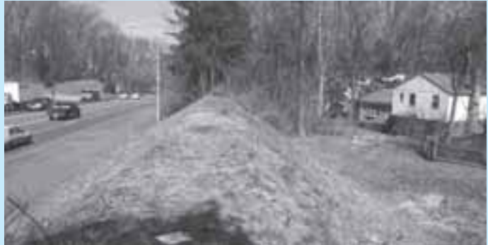
Berm construction is generally preferred by builders.
